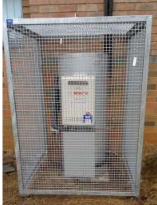
The solar hot water tank with protective cage
